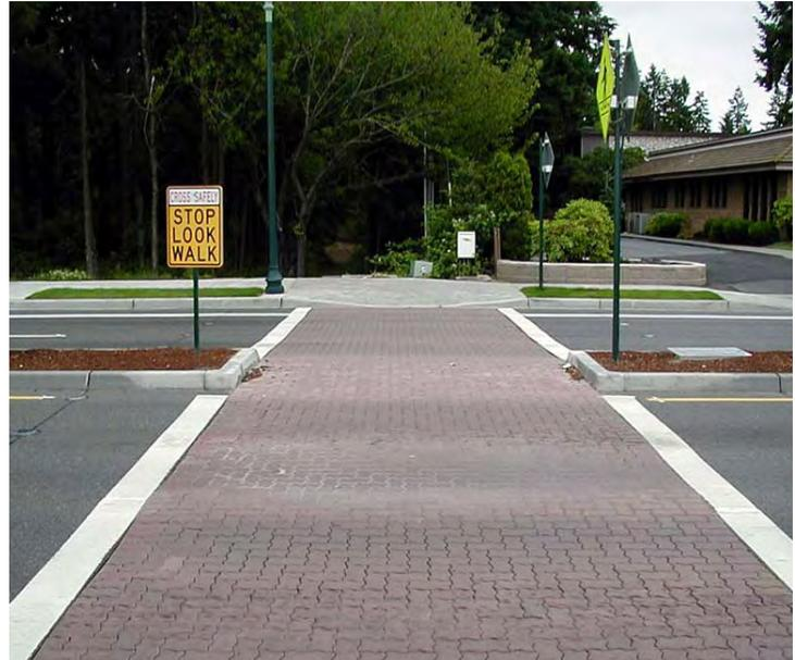
This mid-street, at grade pedestrian crosswalk is the most common type of street crossing. Because of the inherent danger of at-grade crossings, it is imperative that the appropriate signage for drivers and pedestrians is present.
